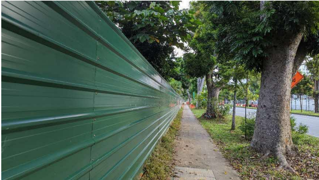
Figure 8.4. Example of the permanent hoarding
